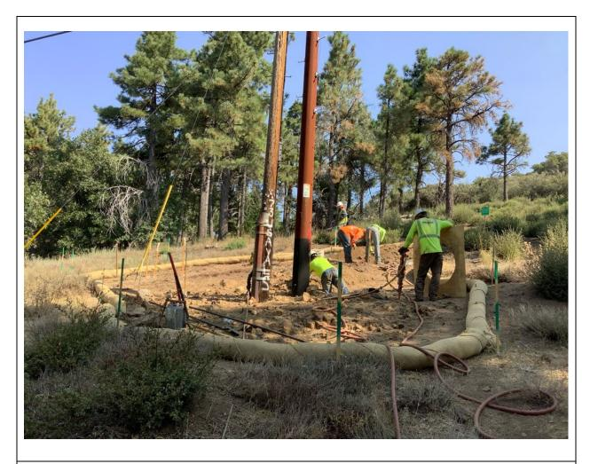
**Photo 2:** A crew was observed digging pole and anchor excavations at Pole P40370 (C 440). Crew members and materials were observed remaining within clearly delineated work limits in accordance with MM BIO-1.
