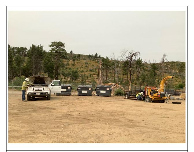
**Photo 5:** A crew was observed conducting vehicle and equipment maintenance at Shrine Camp Staging Yard (C 440). Drip pans were observed under vehicles and equipment during maintenance to prevent leaks or spills from being discharged onto the ground in accordance with the SRNP and MM PHS-2.
