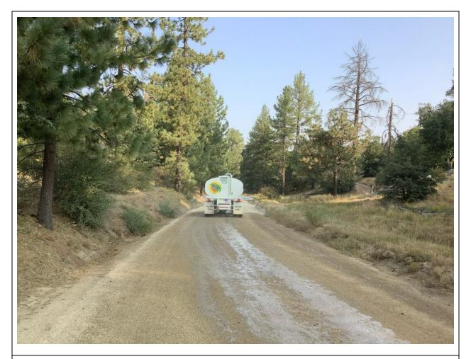
**Photo 1:** A water tender was observed applying water to the surface on Los Huecos Road (C 440) to minimize dust emissions from Project vehicular traffic in accordance with APM AIR-02.
