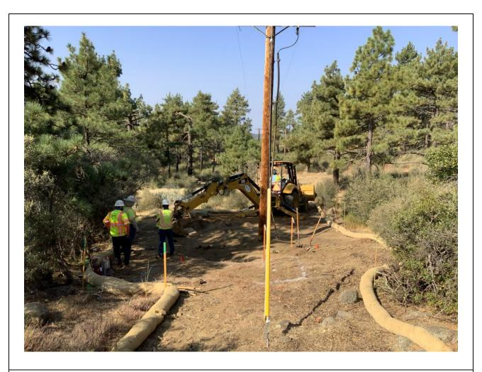
**Photo 6:** A crew was observed excavating a trench for a retaining wall near Pole P40143 (C 440). Site-specific erosion control BMPs were observed in good condition in accordance with the ECP, SWPPP (MM HYD-1 and MM BIO-7), and APM HYD-09.
